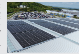
Solar panels at Kota Plant
