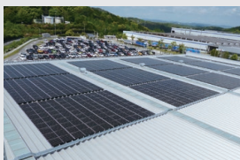
Solar panels at Kota Plant
