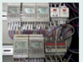
Timer-based controller for air conditioners
